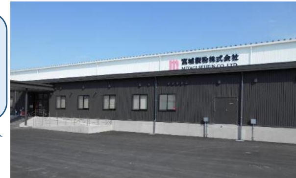
Photo: Exterior view of the new plant
